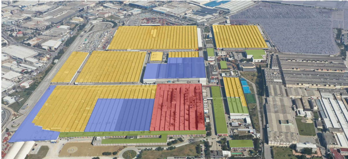
Figure 14. Overview of available surfaces for on-site renewable energy deployment at the TOFAS site.
