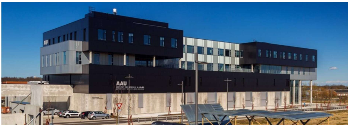
Figure 4. The AAU demo site building in Aalborg, Denmark. Picture: Thomas Pedersen
