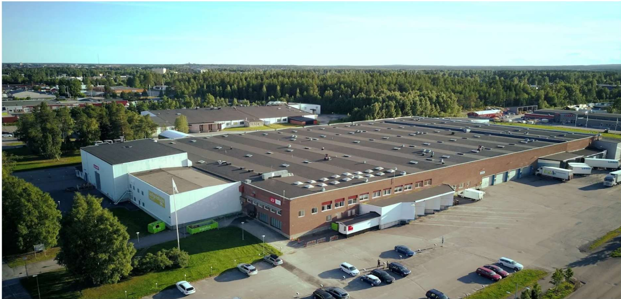
Figure 10. The RISE demo site building in Luleå, Sweden.
