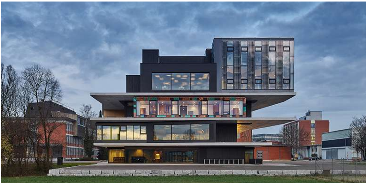
Figure 8. The EMPA demo site building in Dübendorf, Switzerland.
