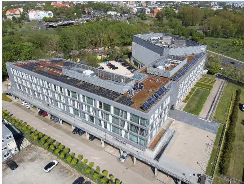
Figure 15. The PSNC demo site building in Poznan, Poland.
