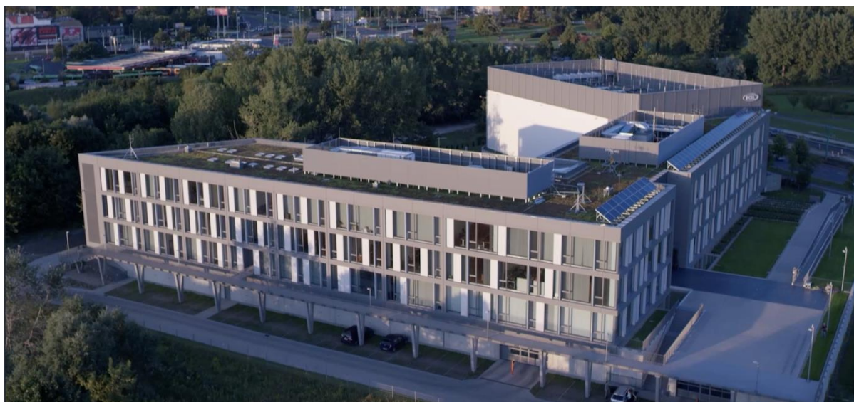
Figure 2.120: Picture of the PSNC pilot building.
