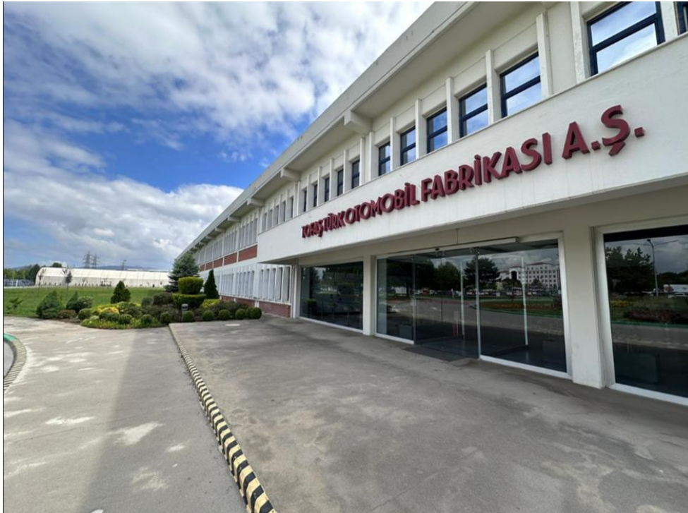
Figure 2.112: Main building of the TOFAS car factory, the image shows the IT office part in the ground floor (see Figure 2.111 for location details).
